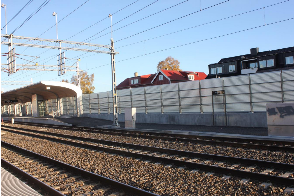
Figure 6B4: Umeå C ,the central train station. Noise barriers have been set up to improve the sound environment for local residents and the cargo railway yard has been moved out of the city.
