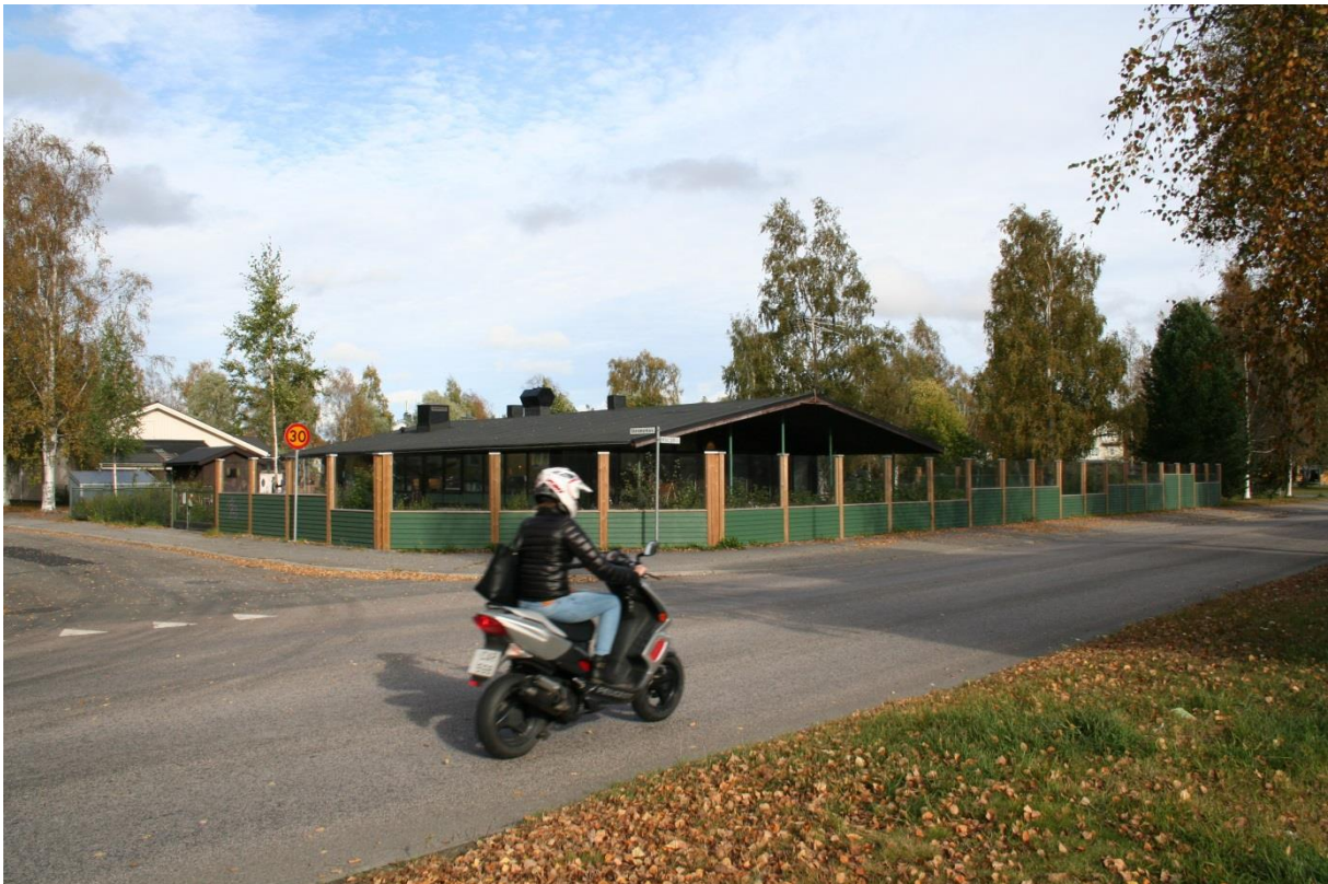
Figure 6B2: Recently built noise barriers (2014), at pre-school in Umeå.
