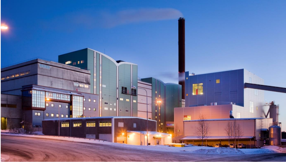
Figure 11B4. Dåva 2 Biofuel combined heat and power plant, opened in 2010.
