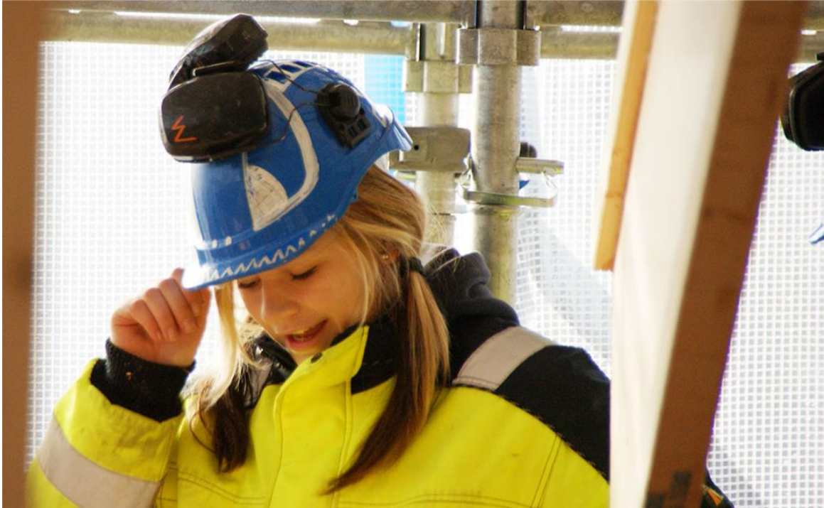
Figure 11B2. Students are building the northern-most single family houses certified to passive house standard. To meet future energy regulations it's important to educate craftsmen with the know-how and workmanship needed to go the extra mile.
